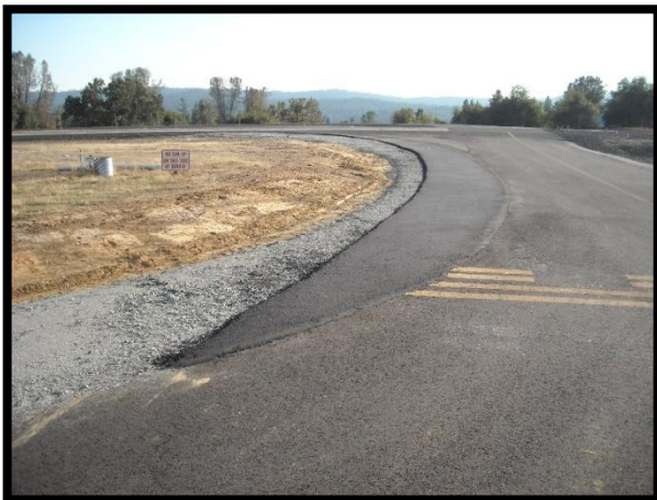
Grading and paving on the Northwest end of the runway
