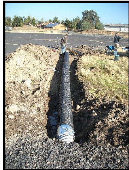
Culvert Installation at the Mid-Field Runway Exit
