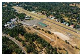
Aerial view-new taxiway
