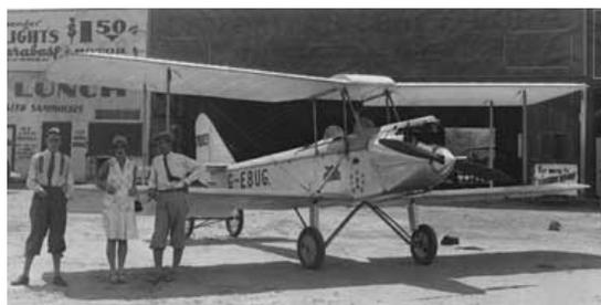
To appreciate the enormity of such a flight, one should read the specs for the aircraft: max speed: 102 mph; cruising speed: 87 mph; climb: 650 fpm; ceiling: 18,000 ft; gas capacity: 35 gal; max range: 400 miles. Aircraft length: 24'3"; height: 8'6"; wingspan: 28'; tare wt: 1130 lbs; max wt: 2002 lbs; present engine: Gypsy II, 120 hp.
